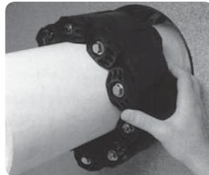
2. Wrap the belt around the pipe and connect the first and last links together.
