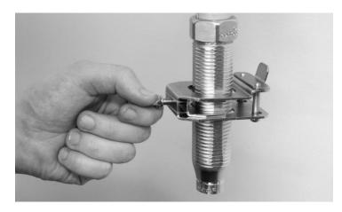
**4.** Apply a non-hardening pipe joint compound or PTFE tape to the male thread of the sprinkler head and install in the Outlet Reducer according to the sprinkler head manufacturer's instructions, using the wrench supplied by the manufacturer.
