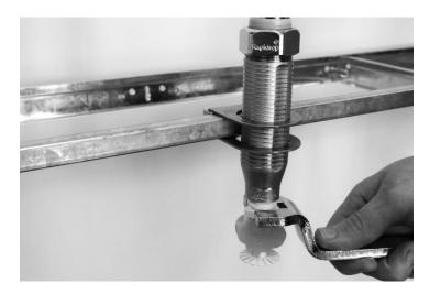
When installing the sprinkler head with a two piece escutcheon, the inner piece should be mounted on the thread of the sprinkler head before attaching to the reducer.
