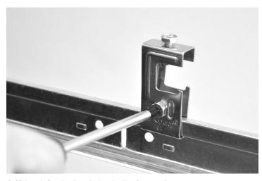
4. Slide A1 Centre Bracket onto the Square Bar.
