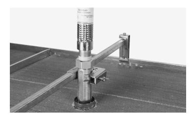
**10.** Adjust height of the Outlet Reducer until desired location of the sprinkler is achieved. Firmly secure the Centre Bracket by tightening the wing bolt to a torque of 5 Nm/4 ft-lbs).
