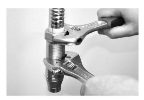
3. Remove plastic Protecting Cap from the other end of the flexible hose, check that the black rubber Seal is in place and connect that end to the inlet nipple on the range pipe and tighten the nut to a torque of 20 Nm/15 ft-lbs).
