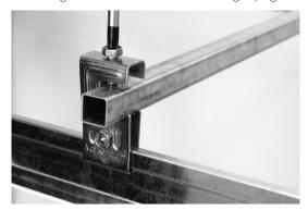
Adjust location of the centre bracket and the side B brackets until desired location of the outlet reducer is achieved. Firmly secure the side B brackets by tightening the screws to a torque of 5 Nm/4 ft-lbs.
