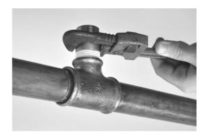
Remove plastic Protecting Cap from one end of the flexible hose, check that the black rubber seal is in place and connect the Outlet Reducer (M33 x 1.5 thread end) to that end. To prevent reducer from turning, securely hold in place whilst tightening the hose nut. Tighten to a torque of 20 Nm/15 ft-lbs. Do not exceed the specified torque.
