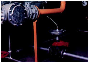
The combination of the Continuous desalting valve\* and the Blowdown valve for bleeding dirt and sludge\* is essential for optimizing the boiler's efficiency, and include its maximum security and availability.
